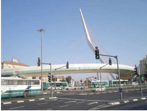
Fig. 2a: The 'Chords Bridge'
